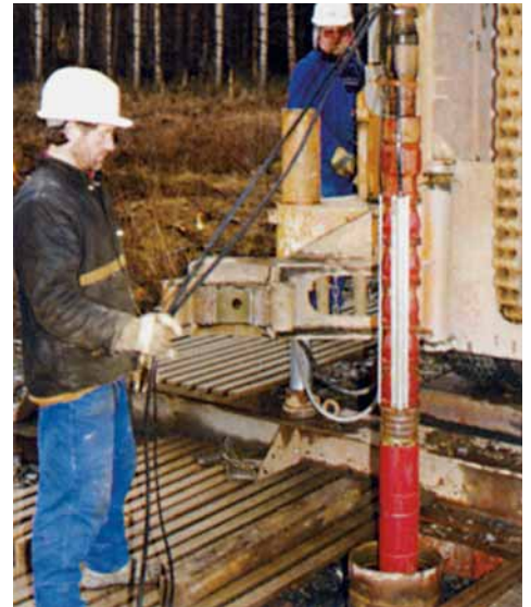
Long-life borehole pumps are available for dewatering applications: up to 600 GPM at 1,360' TDH
